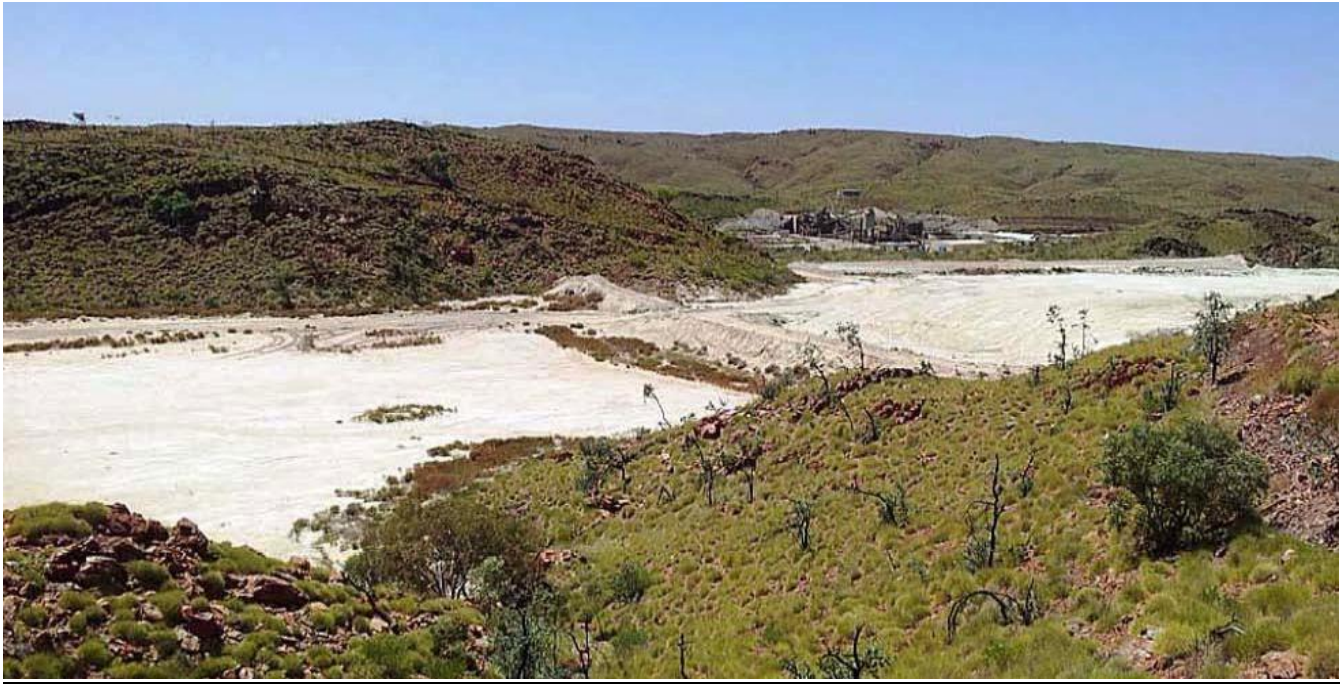
Figure 18: Bamboo Creek Tailings Storage with Bamboo Creek Processing Plant in background
