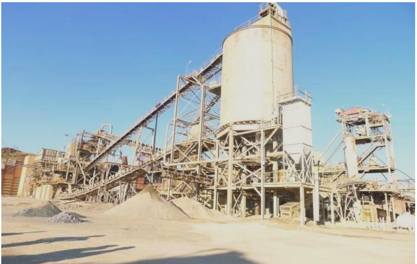
Figure 17: Bamboo Creek Processing Plant
