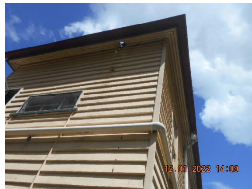
Missing downpipe
