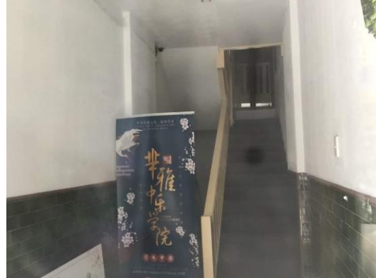
Staircase to first floor
