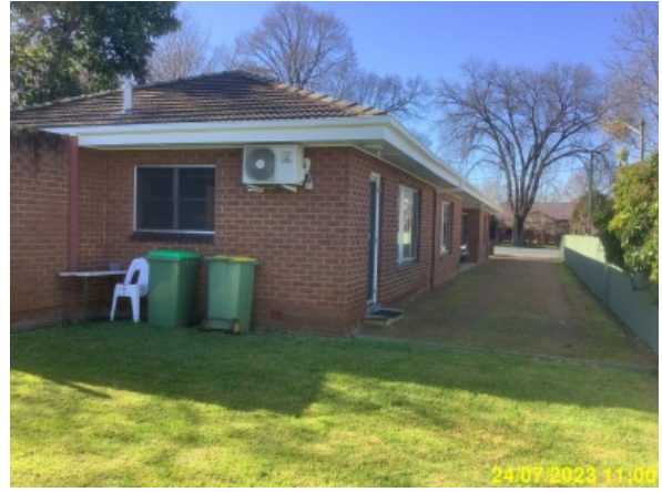
Description: Rear Elevation
