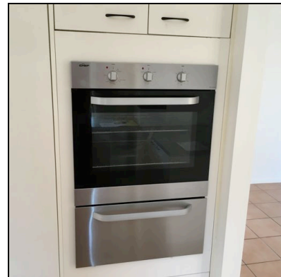
Photo No: 004 Oven
