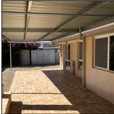
Photo No: 007 Patio Area
