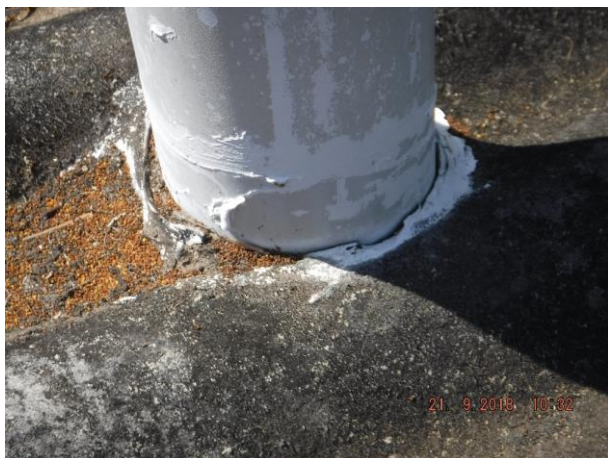
South west vent pipe has no flashing fitted or PVC collar and carport roof to dwelling junction is not flash sealed Refer 3.02 and 3.01
