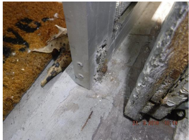
Unit 2 lounge west window has fibro used to galleries instead of glass and unit 2 fly screen door to entry is heavily corroded – Refer 1.06 and 1.07
