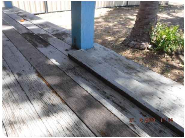
Front balcony handrail newel posts are loose to subfloor timbers and has some loose floor boards – Refer 2.11
