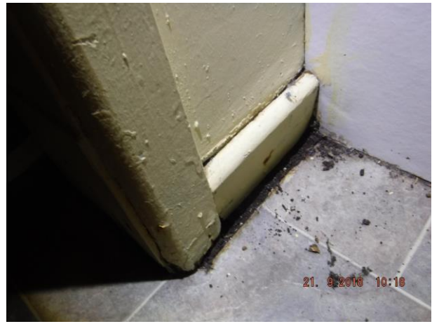
Unit 2 shower north wall has previous moisture damage and patch repair – Refer 1.02
