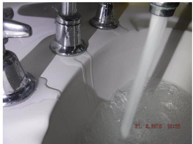
Unit 2 laminated splashback to kitchen is loose to wall linings and unit 2 vanity taps and spout are all leaking Refer 1.09(d) and 1.10(d)
