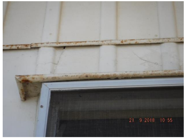
Exterior asbestos wall claddings are significantly cracked and broken – Refer 2.03
