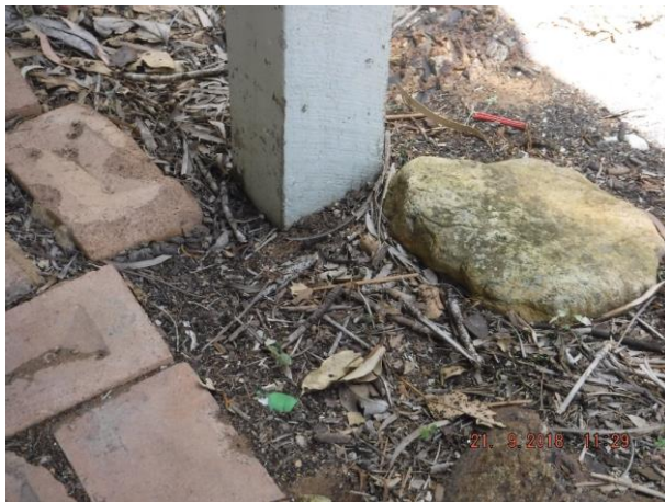
Unit 2 carport timber support post encased in ground and corroded roof sheeting – Refer 6.01
