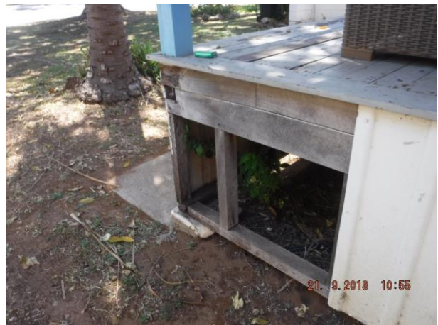
Exterior asbestos wall claddings are significantly cracked and broken and some missing sheeting – Refer 2.03
