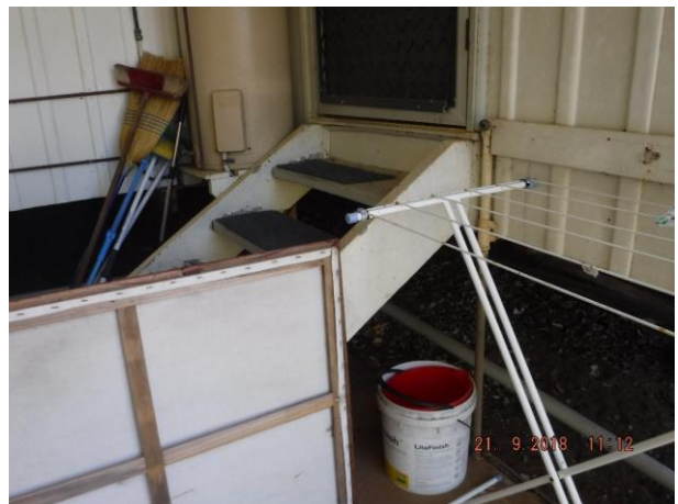
Unit 2 front timber stairs bottom 2 nd tread has significant wood decay and unit 1 rear timber stairs has no handrail fitted to outside of stairs – Refer 2.10
