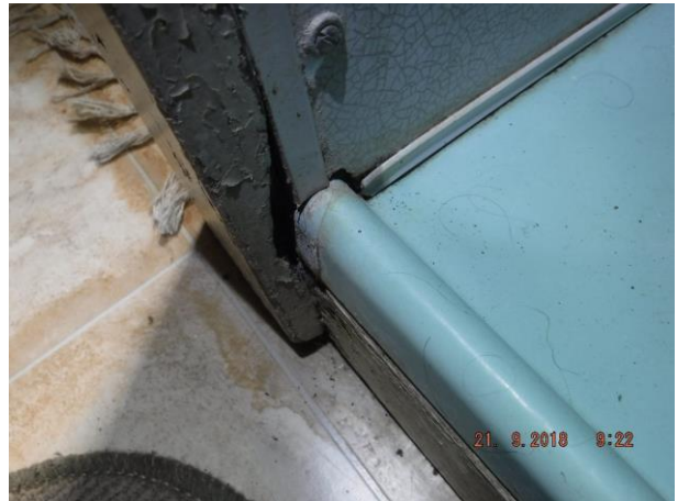
Unit 1 shower walls have moisture damage – Refer 1.02
