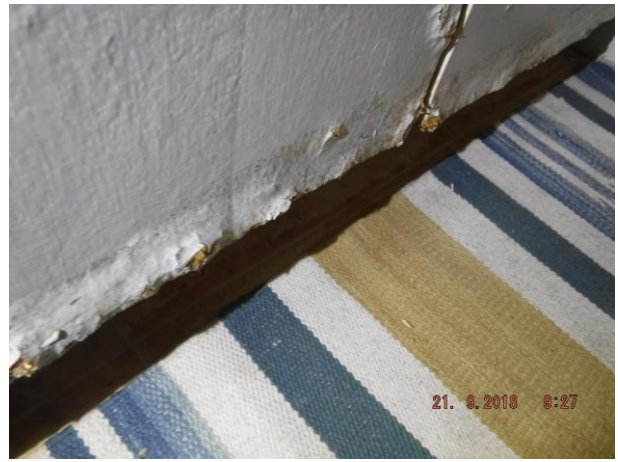
Unit 1 shower cubicle lami panel wall linings are loose to shower tray recess and unit 1 vanity has delaminating shelving and doors – Refer 1.10 (f) and (h)
