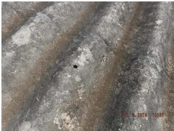
Asbestos roof sheeting and flashings have missing fixings and asbestos guttering is full of leaf debris – Refer 3.01 and 3.04
