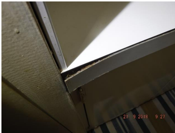
Unit 1 vanity has delaminating bench top edge strip and unit 1 laundry tub cold tap has leaking tap fitting and tap washer Refer 1.10(h) and 1.11(b)
