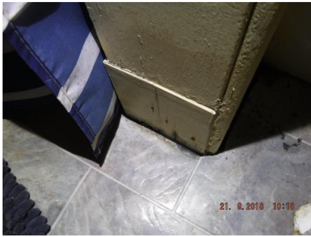
Unit 2 shower north wall has previous moisture damage and patch repair – Refer 1.02
