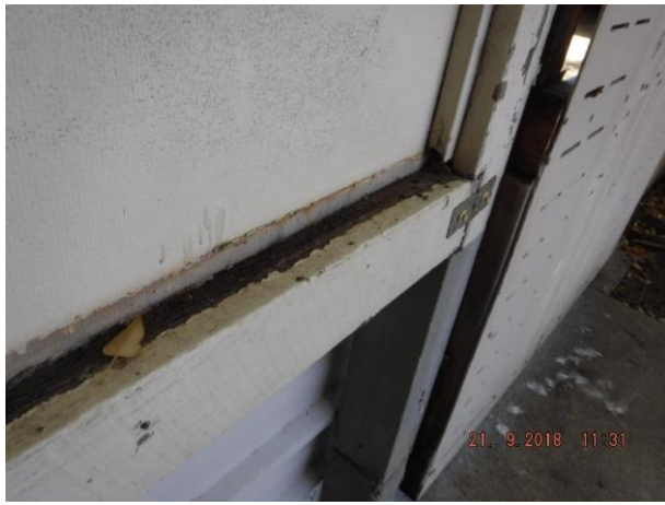
Laundry separating wall has had previous minor termite entry and damage and rear shed has defective sheeting Refer 5.03 and 6.04
