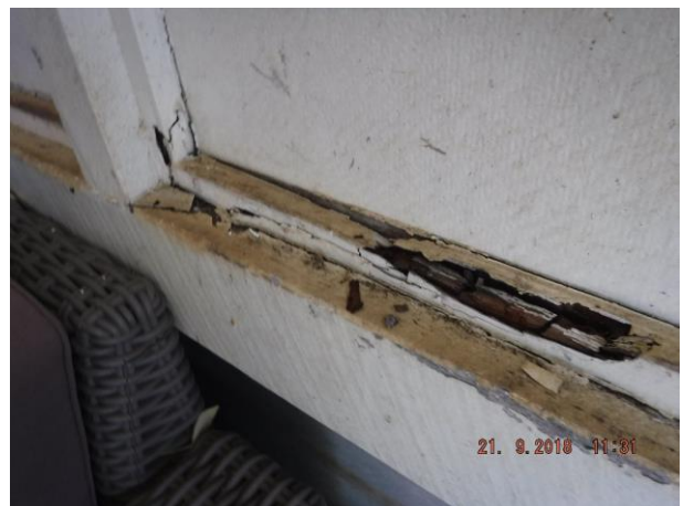
Defective brick paved floor to unit 2 carport and laundry separating wall has had previous minor termite entry and damage Refer 6.01 and 5.03
