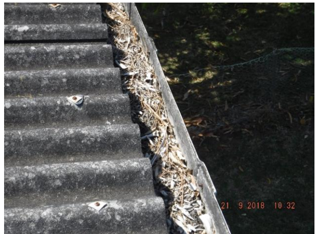
Asbestos roof sheeting and flashings have missing fixings and asbestos guttering is full of leaf debris – Refer 3.01 and 3.04
