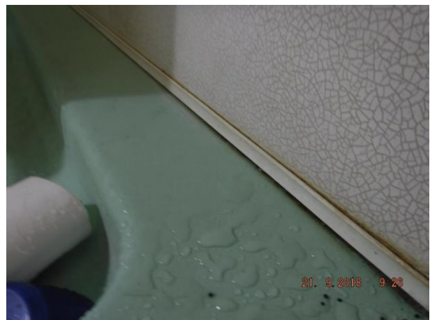
Unit 1 toilet has deteriorated and leaking cistern to pan rubber connector and unit 1 shower cubicle lami panel wall linings are loose to shower tray recess – Refer 1.10(d) and (f)
