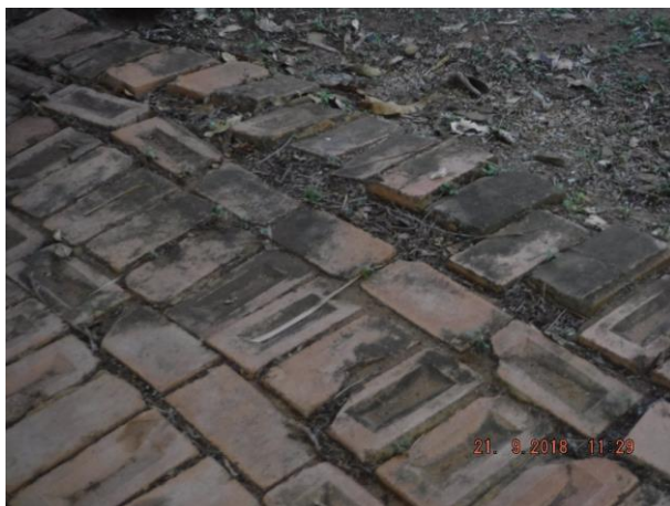
Defective brick paved floor to unit 2 carport and laundry separating wall has had previous minor termite entry and damage Refer 6.01 and 5.03
