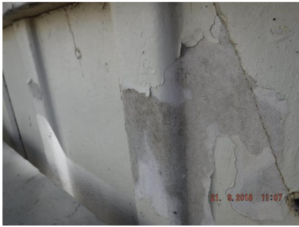
Exterior of duplex has peeling paint from wall claddings, balcony timbers, doors and trims – Refer 2.08
