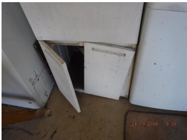
Unit 1 laundry tub cabinet has defective right door and unit 2 lounge and kitchen ceiling has peeling paint Refer 1.11(c) and 1.01
