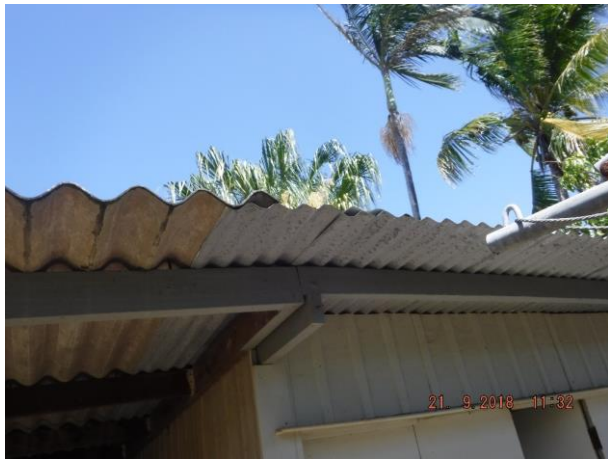
Rear shed has defectively lapped sheeting and timber frame encased inground allowing vermin entry – Refer 6.04
