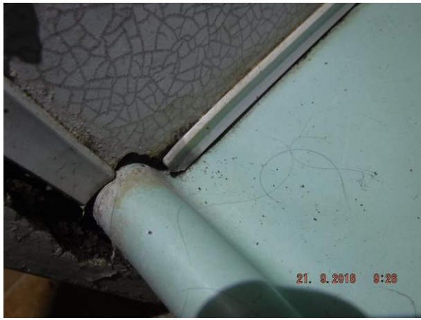
Unit 1 shower cubicle lami panel wall linings are loose to shower tray recess and unit 1 vanity has delaminating shelving and doors – Refer 1.10 (f) and (h)
