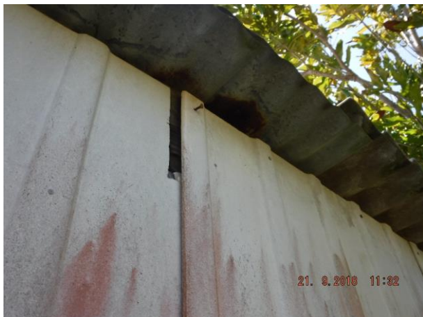
Rear shed has defective sheeting – Refer 6.04
