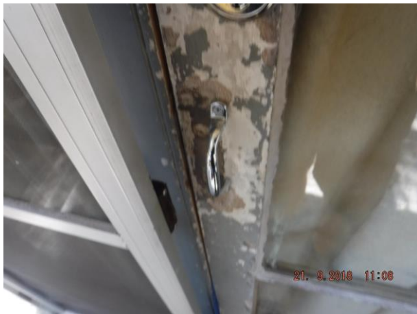
Exterior of duplex has peeling paint from wall claddings, balcony timbers, doors and trims and unit 2 front timber stairs bottom tread has significant wood decay – Refer 2.08 and 2.10
