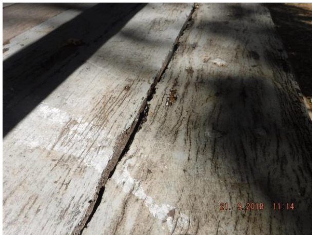
Wood decay to front balcony floor boards and concrete stump has significantly cracked from corroded reinforcing Refer 2.11 and 5.01
