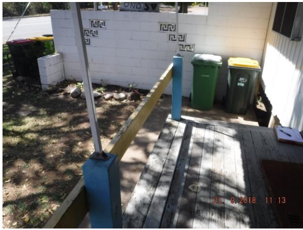
Front balcony handrail newel posts are loose to subfloor timbers and has some loose floor boards – Refer 2.11
