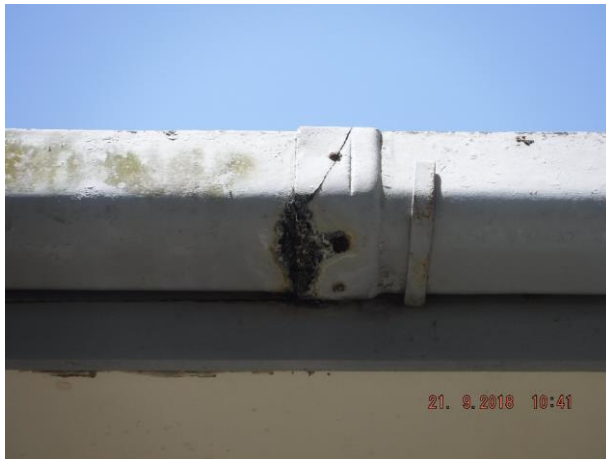
Front and rear gutter joints are cracked and leaking – Refer 3.04
