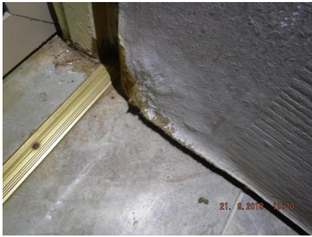
Unit 2 rear entry timber door is an internal use door and has moisture damage and unit 2 toilet door is delaminated Refer 1.07
