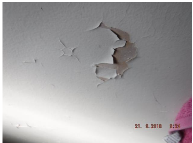
Peeling paint to unit 1 walls – Refer 1.02
