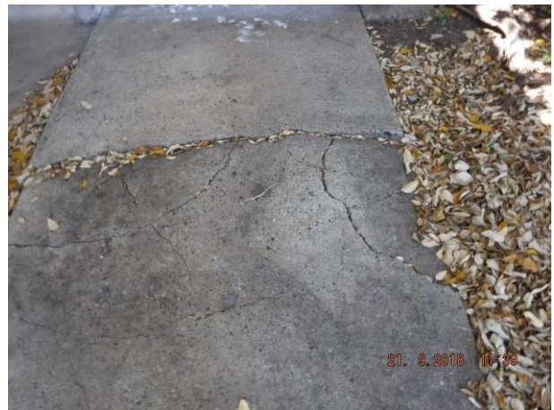
Rear shed has previous termite damage and rear concrete path to unit 1 has some concrete cracking and subsidence Refer 6.04 and 6.06
