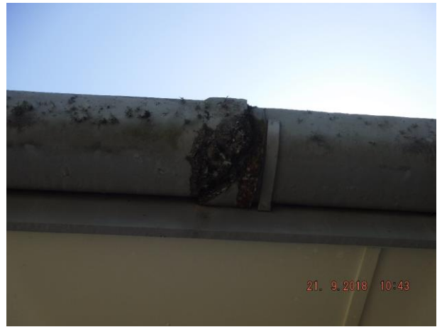
Front and rear gutter joints are cracked and leaking – Refer 3.04
