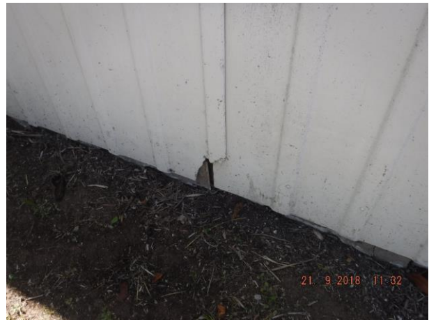
Laundry separating wall has had previous minor termite entry and damage and rear shed has defective sheeting Refer 5.03 and 6.04
