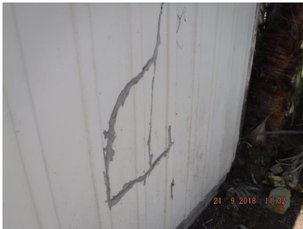
Rear shed has defective sheeting – Refer 6.04
