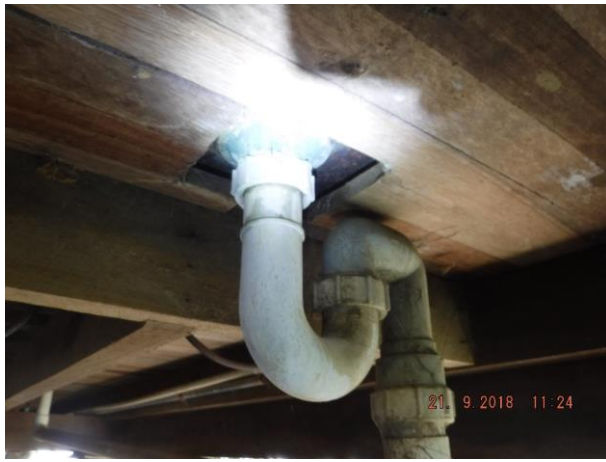
Unit 1 shower waste trap is leaking and unit 2 carport timber support posts not adequately supported – Refer 5.01 and 6.01
