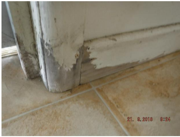
Peeling paint to unit 1 and unit 1 kitchen bench top has gap between top and skirt tile junction – Refer 1.02 and 1.09(a)
