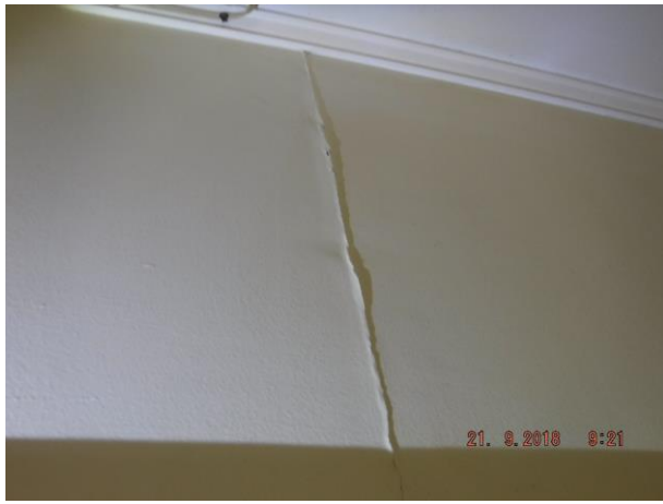
Unit 1 wall linings have some movement cracking – Refer 1.02
