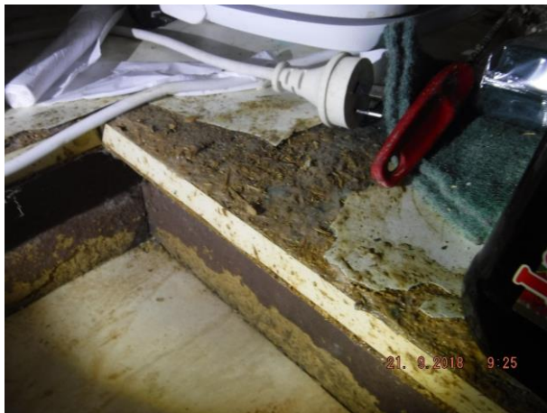
Unit 1 kitchen cabinetry is badly deteriorated and moisture damaged – Refer 1.09(b)
