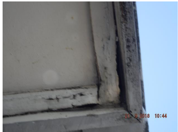
Rear downpipe is missing and south west corner eave has wood decayed timber cover strips – Refer 3.04 and 3.05
