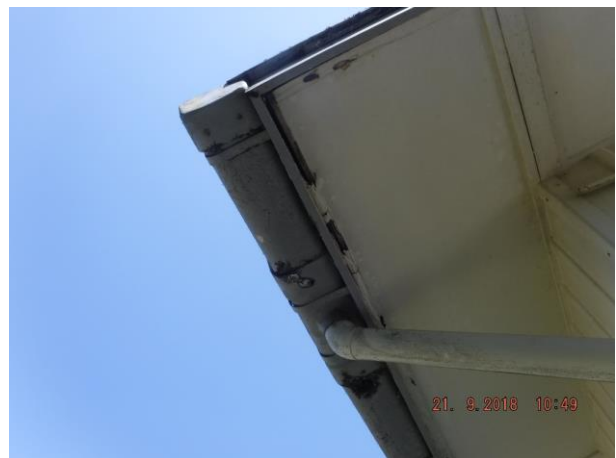
Front east side downpipe is starting to undermine concrete stump footing and rear south east eave is moisture damaged – Refer 3.04 and 3.05
