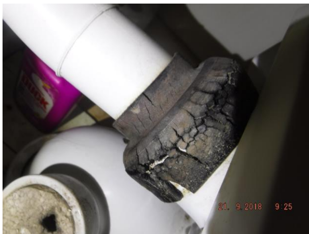
Unit 1 toilet has deteriorated and leaking cistern to pan rubber connector and unit 1 shower cubicle lami panel wall linings are loose to shower tray recess – Refer 1.10(d) and (f)
