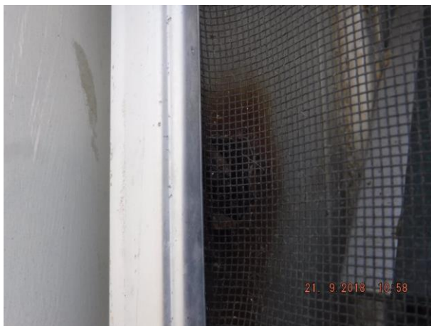
Exterior timber boxed fly screen frames have some wood decay and loose and corroded fixings – Refer 2.07
