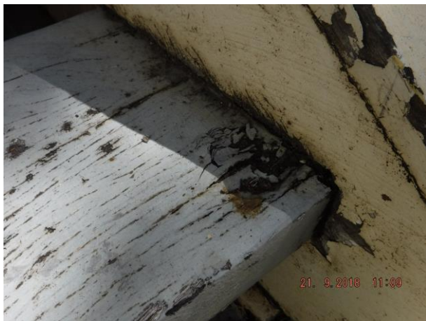
Unit 2 front timber stairs bottom 2 nd tread has significant wood decay and unit 1 rear timber stairs has no handrail fitted to outside of stairs – Refer 2.10
