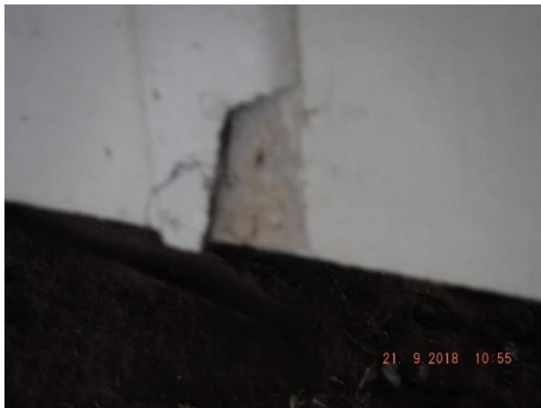
Exterior asbestos wall claddings are significantly cracked and broken and some missing sheeting – Refer 2.03
