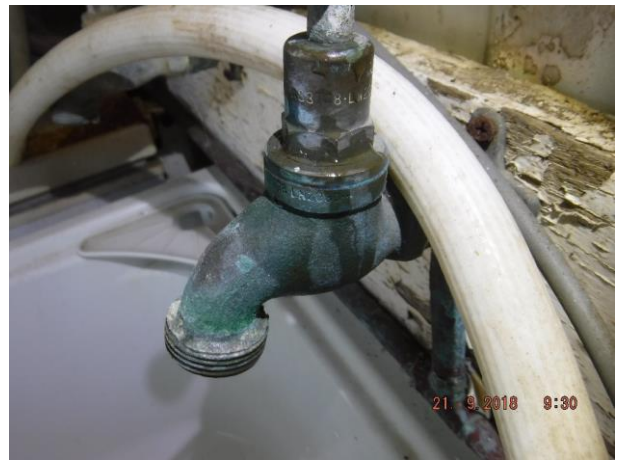
Unit 1 vanity has delaminating bench top edge strip and unit 1 laundry tub cold tap has leaking tap fitting and tap washer Refer 1.10(h) and 1.11(b)
