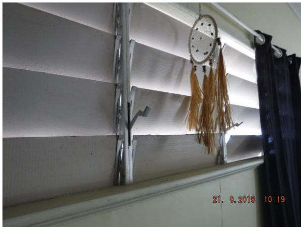
Unit 2 lounge west window has fibro used to galleries instead of glass and unit 2 fly screen door to entry is heavily corroded – Refer 1.06 and 1.07
