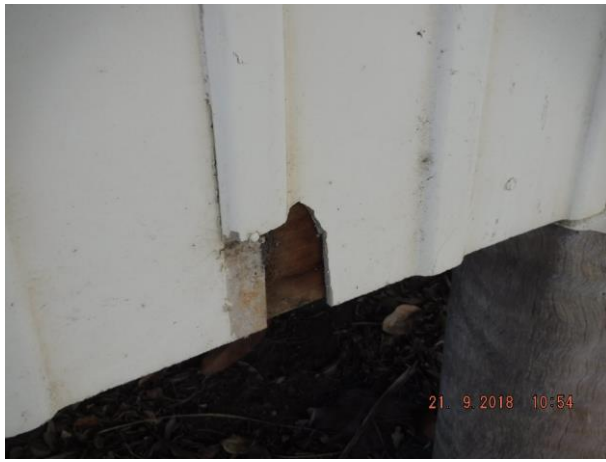
Exterior asbestos wall claddings are significantly cracked and broken – Refer 2.03
