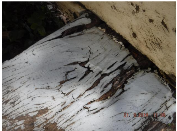
Exterior of duplex has peeling paint from wall claddings, balcony timbers, doors and trims and unit 2 front timber stairs bottom tread has significant wood decay – Refer 2.08 and 2.10
