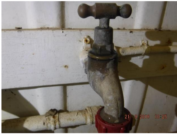
Unit 2 hot water tap is leaking and asbestos roof sheeting and flashings have loose fixings – Refer 1.11(b) and 3.01
