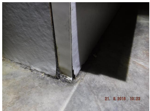
Unit 2 vanity laminated splashback is defective and unit 2 vanity is significantly moisture damaged at base of cabinet Refer 1.10(e) and (h)
