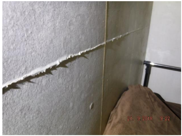
Unit 1 wall linings have some movement cracking – Refer 1.02
