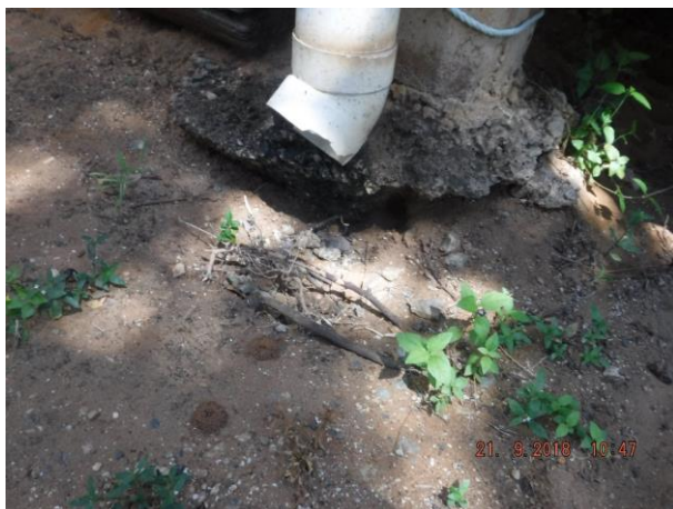
Front east side downpipe is starting to undermine concrete stump footing and rear south east eave is moisture damaged – Refer 3.04 and 3.05
