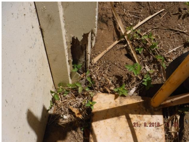
Rear shed has previous termite damage and rear concrete path to unit 1 has some concrete cracking and subsidence Refer 6.04 and 6.06
