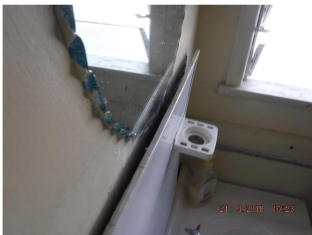
Unit 2 vanity laminated splashback is defective and unit 2 vanity is significantly moisture damaged at base of cabinet Refer 1.10(e) and (h)
