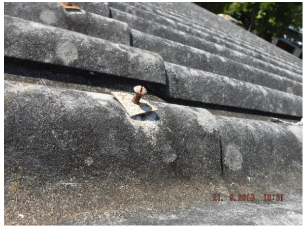
Unit 2 hot water tap is leaking and asbestos roof sheeting and flashings have loose fixings – Refer 1.11(b) and 3.01
