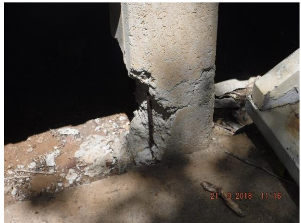
Wood decay to front balcony floor boards and concrete stump has significantly cracked from corroded reinforcing Refer 2.11 and 5.01
