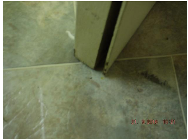
Unit 2 rear entry timber door is an internal use door and has moisture damage and unit 2 toilet door is delaminated Refer 1.07
