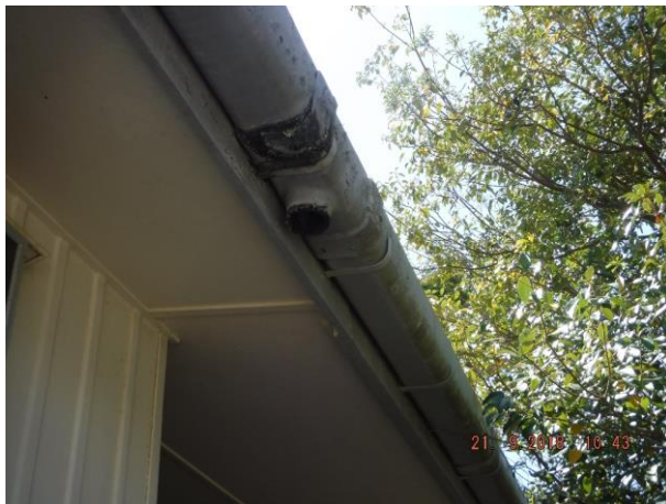
Rear downpipe is missing and south west corner eave has wood decayed timber cover strips – Refer 3.04 and 3.05
