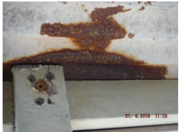
Unit 2 carport timber support post encased in ground and corroded roof sheeting – Refer 6.01
