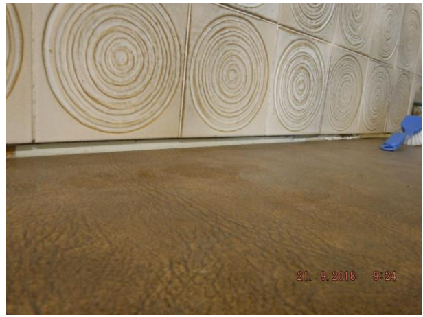
Peeling paint to unit 1 and unit 1 kitchen bench top has gap between top and skirt tile junction – Refer 1.02 and 1.09(a)
