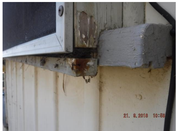
Exterior timber boxed fly screen frames have some wood decay and loose and corroded fixings – Refer 2.07
