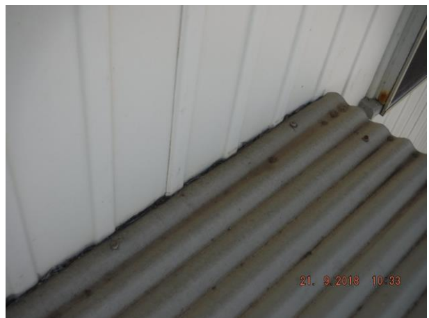
South west vent pipe has no flashing fitted or PVC collar and carport roof to dwelling junction is not flash sealed Refer 3.02 and 3.01
