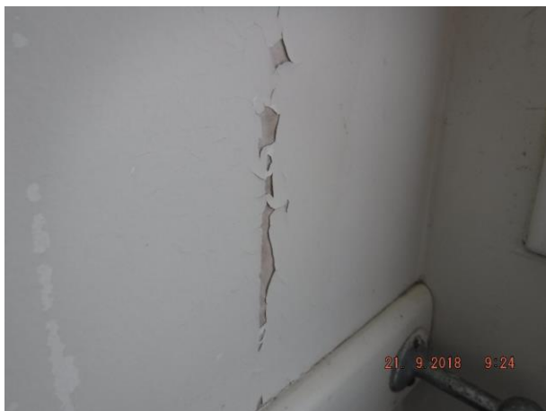
Peeling paint to unit 1 walls – Refer 1.02
