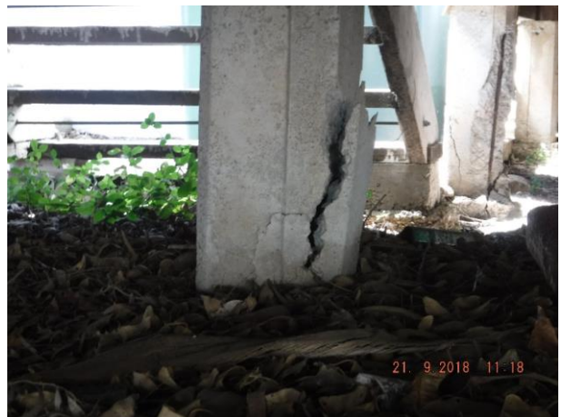
Broken asbestos to underfloor and concrete stump has significantly cracked from corroded reinforcing – Refer 5.01
