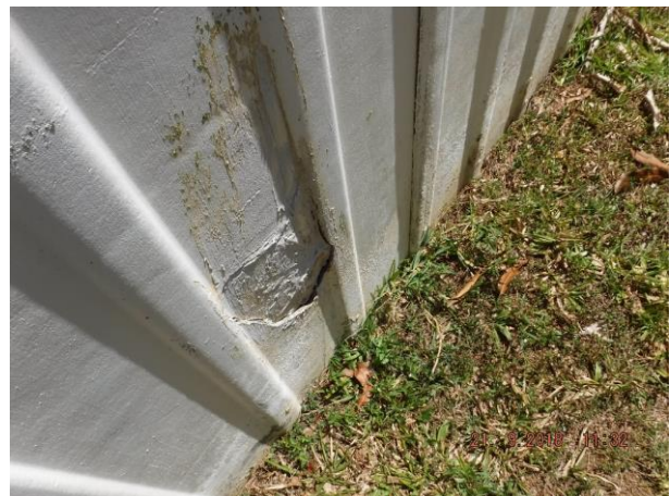
Rear shed has defective sheeting – Refer 6.04
