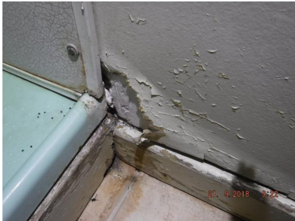
Unit 1 shower walls have moisture damage – Refer 1.02
