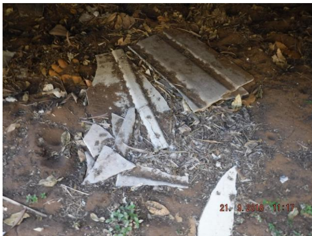
Broken asbestos to underfloor and concrete stump has significantly cracked from corroded reinforcing – Refer 5.01
