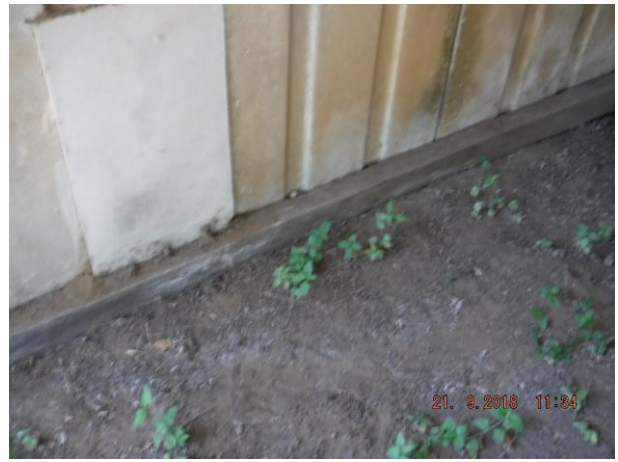
Rear shed has defectively lapped sheeting and timber frame encased inground allowing vermin entry – Refer 6.04
