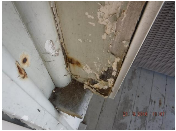
Exterior of duplex has peeling paint from wall claddings, balcony timbers, doors and trims – Refer 2.08
