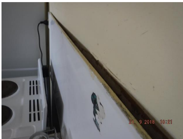
Unit 2 laminated splashback to kitchen is loose to wall linings and unit 2 vanity taps and spout are all leaking Refer 1.09(d) and 1.10(d)
