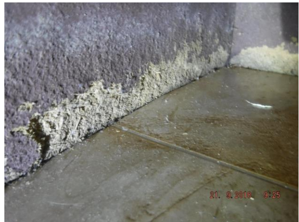
Unit 1 kitchen cabinetry is badly deteriorated and moisture damaged – Refer 1.09(b)
