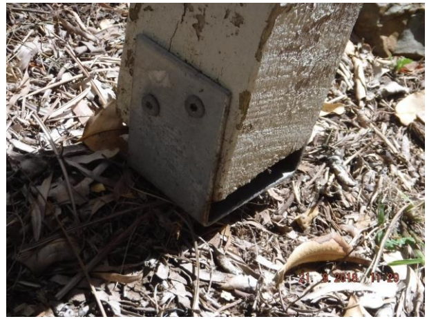
Unit 1 shower waste trap is leaking and unit 2 carport timber support posts not adequately supported – Refer 5.01 and 6.01
