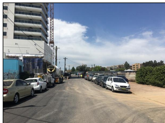
Second Avenue – North Westerly aspect
