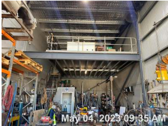
Internal warehouse & mezzanine
