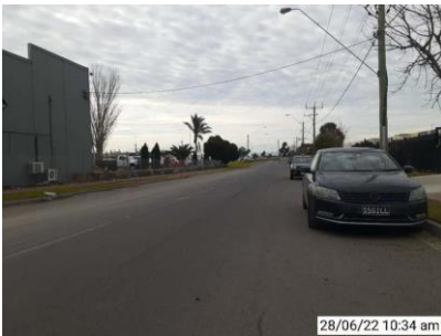
Cooper Street Eastbound
