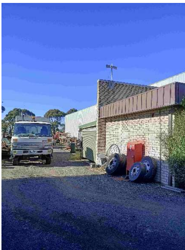
Side of warehouse Lot 38
