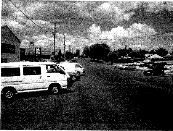
View south along Fitzroy Street
