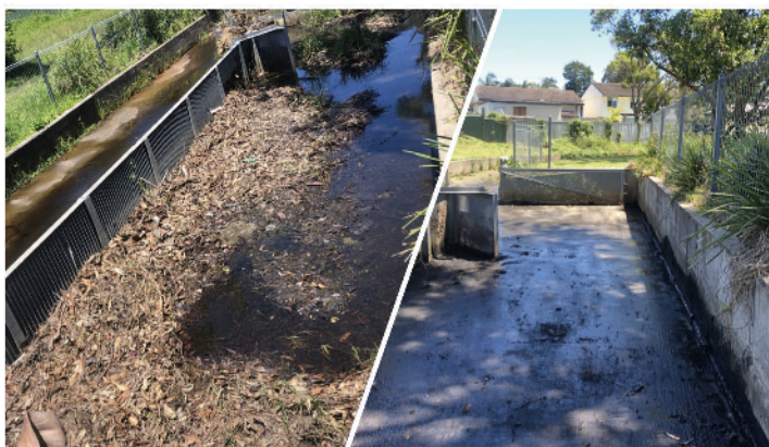
Spring Valley GPT before and after cleaning
