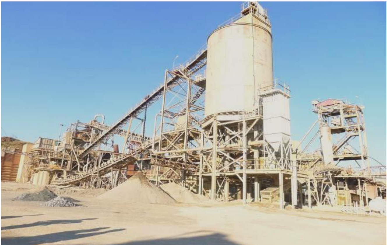
Figure 20: Bamboo Creek Processing Plant
