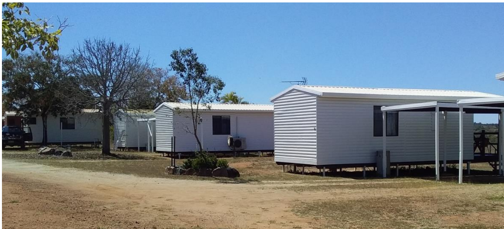
Figure 13(b): Refurbished accommodation cabins at Top Camp
