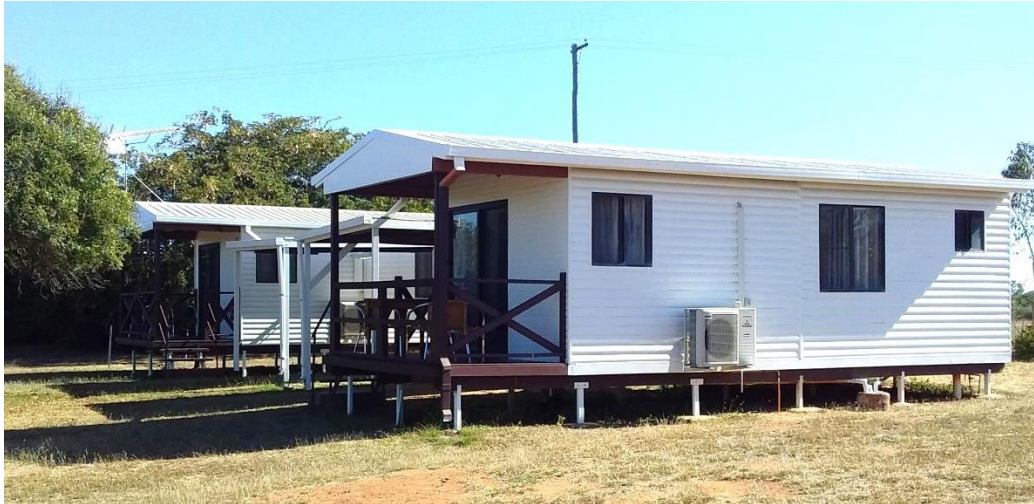
Figure 13(a): Refurbished accommodation cabins at Top Camp
