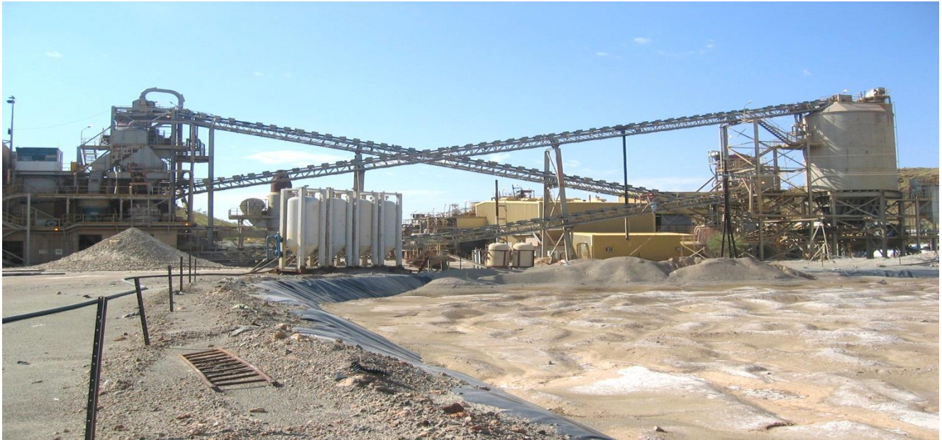
Figure 21: Bamboo Creek Processing Plant
