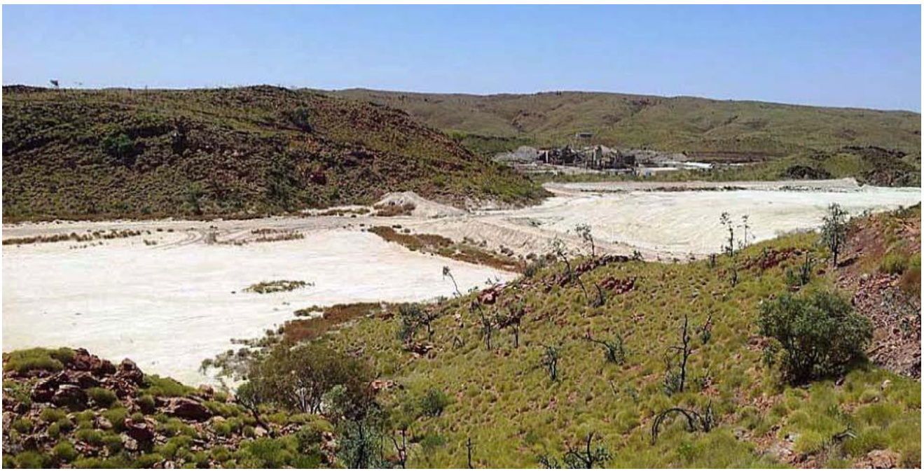
Figure 22: Bamboo Creek Tailings Storage with Bamboo Creek Processing Plant in background
