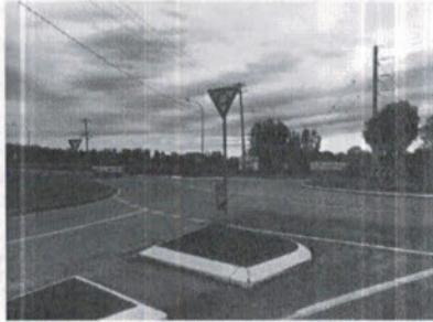
Main roundabout at intersection of Tamarind Rd and Ferngrove Dr
