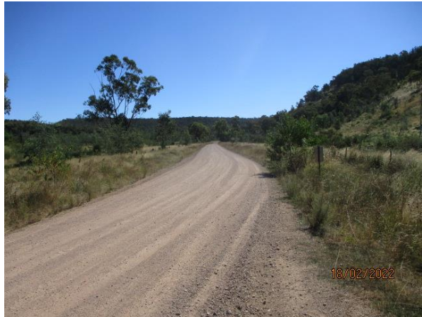
View south-west along Berryrennie Road
