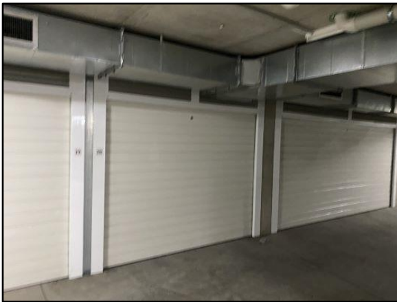
Basement lock up garage
