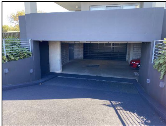
Common access from Quarry Street
