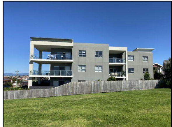
Northern elevation of complex
