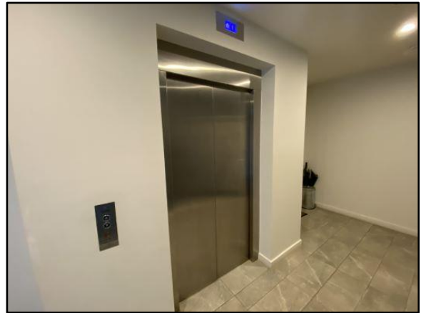
Common lift access
