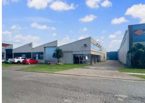
1/360 FISON AVENUE, EAGLE FARM
